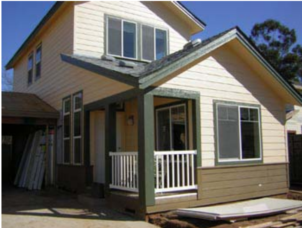
A manufactured home nearly installed in Brotherton Square.
