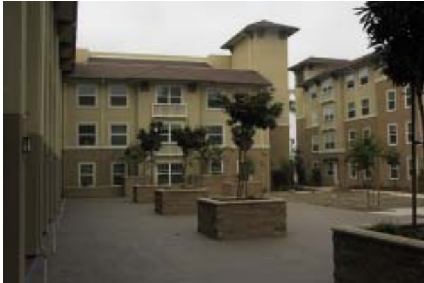
Las Brisas after redevelopment.
